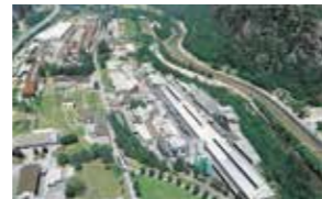
Bodio, Switzerland Graphitization and processing of synthetic graphite, manufacturing of water-based dispersions, processing of natural graphite and coke, and manufacturing and processing of silicon carbide
